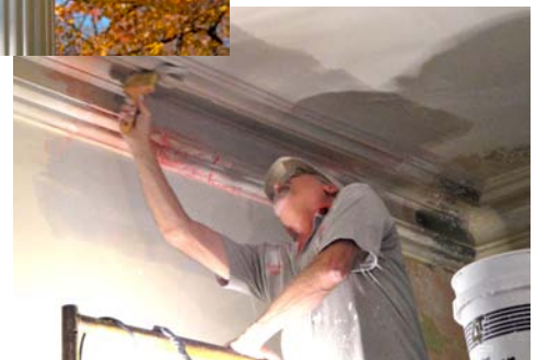
Dallas Schrock of Schrock Plaster Co. repairs plaster moulding.
