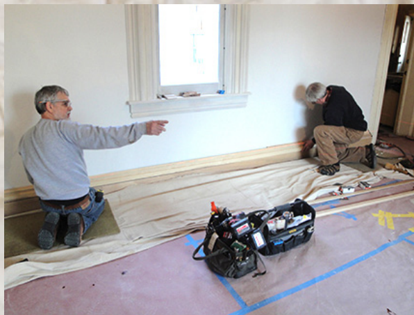
Verlin Miller and Bruce Gowdy install restored baseboards at Havilah Beardsley House
